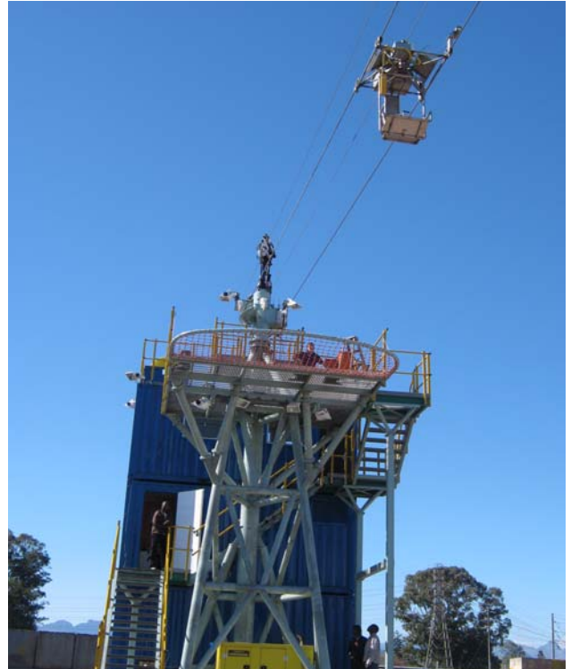
THE AERIAL ROPEWAY SYSTEM DURING COMMISSIONING IN CAPE TOWN IN AUGUST 2010.
