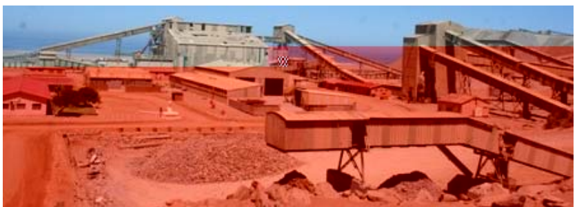
NUMBER 3 TREATMENT PLANT COMPLEX IN SOUTHERN COASTAL MINE
