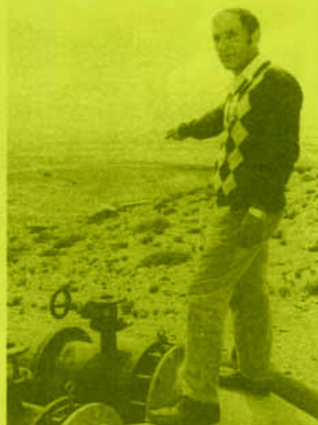
Standing at the reservoirs on Swartkops, Plumber Shop foreman, Hennie van Tonder points to the deep channel in the faraway Orange River.
